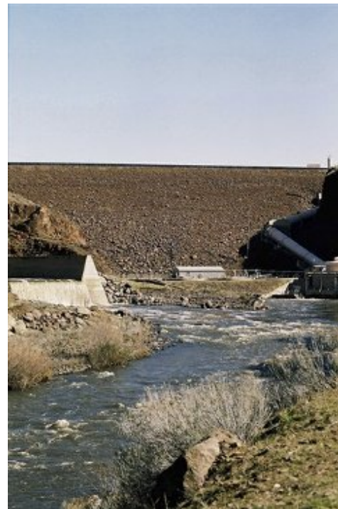
Figure 6 - Irongate Dam in Northern California
